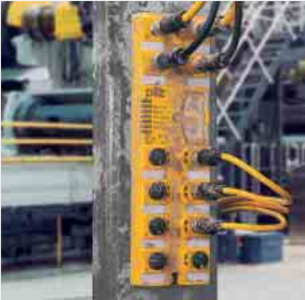
PSS67 – Resistant to dirt and water in accordance with IP67.
